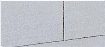
CCS Reveal SB 1 for fine exposure depth of 0.5 to 1.0mm
